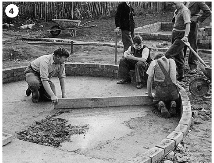
Pic 4: Building an ornamental bridge in the gardens of the First School in around 1957 proved to be the start of a successful career for Len Jarvis (left), starting out in what was to become his trade for the rest of his working life, as a master builder. Len specialised in renovating old buildings and was highly respected in the region.
