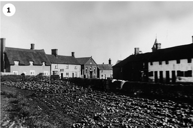
Pic 1: Green End, the cottages and the Spotted Cow public house – long since demolished but the Chapel still stands.
