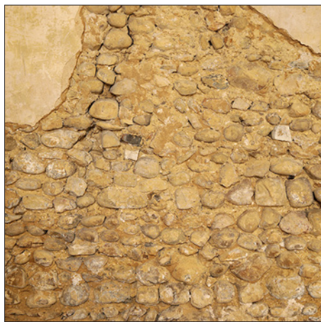
The walls of St Denis were made from field stones, the size of cobbles, in the 12 th century. Those in the nave are still in fine condition.
