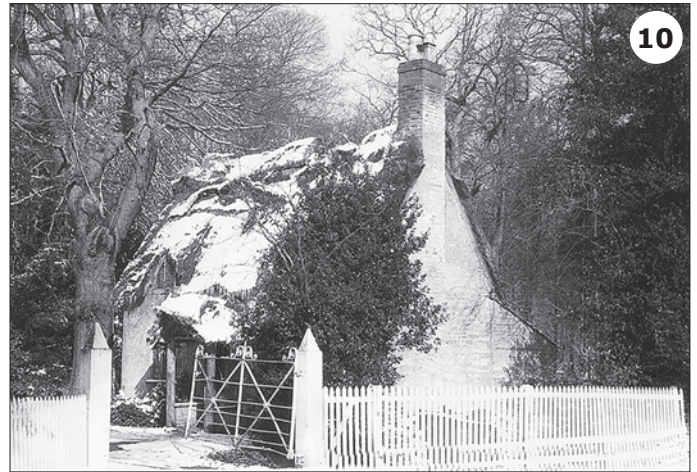
Pic 10: This thatched cottage on the edge of Woodbury Estate, which still stands today, underwent an extensive refurbishment in the early 1970's just after this picture was taken. The thatch on the roof was in very bad condition and a lot of damage was done that winter because of bad weather.
