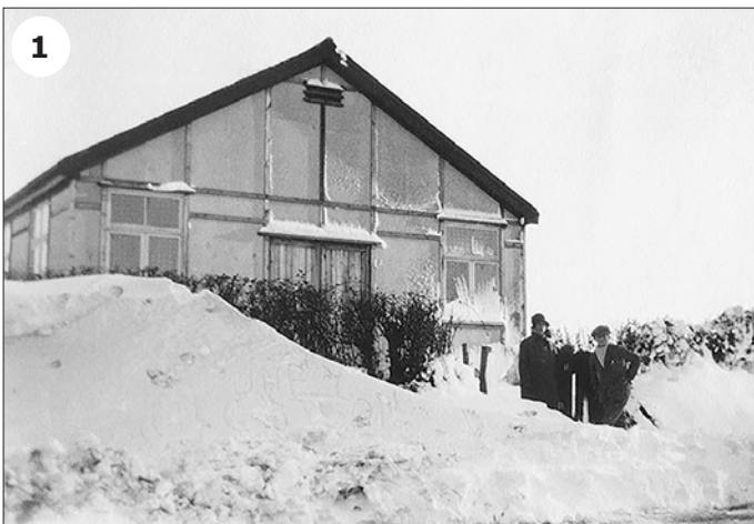
Pic 1: The Women's Institute building in Waresley Road, winter 1927. The deep snow drift being cleared by the Ellis family.
