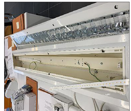
Fluorescent fittings being converted to LED.
